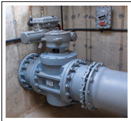
Cam-Centric® Plug Valve with motor actuator
