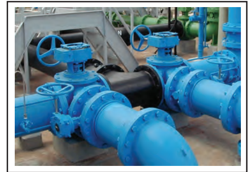
3-Way Cam-Centric® Plug Valves with worm gear actuators
